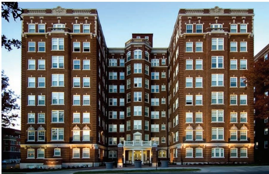
Georgian Court Apartments, Kansas City, Missouri
