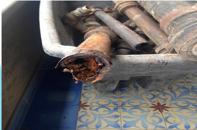
Original pipe – J-wing
