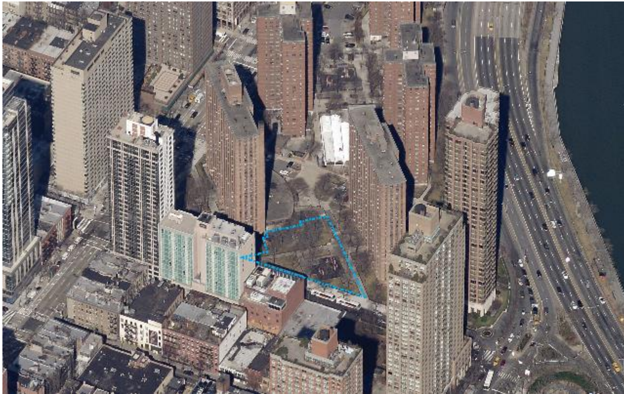
Aerial Image from South
