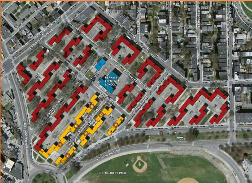
site aerial pre-construction
