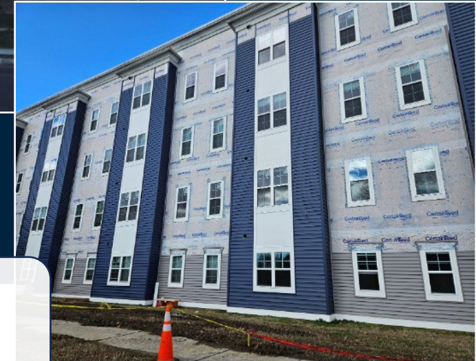
Owens Queen Manor under construction
