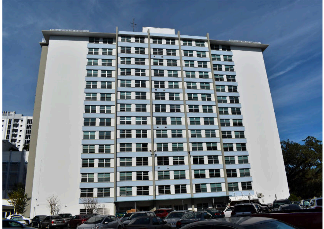
Baptist Terrace Apartments, South Facade, 2023
