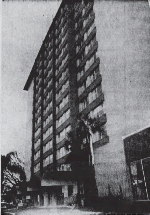
Baptist Terrace upon completion. Source: Orlando Sentinel, March 8, 1970.
