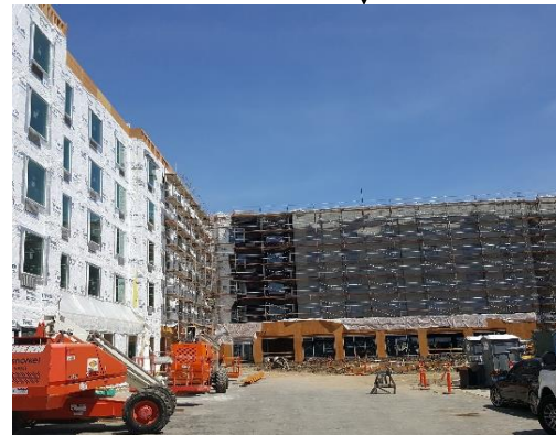
4. Siding & Roofing Outside, MEP & Finish Inside
