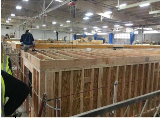
1. Modules Built in Factory
