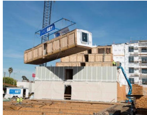
3. Craned and Connected
