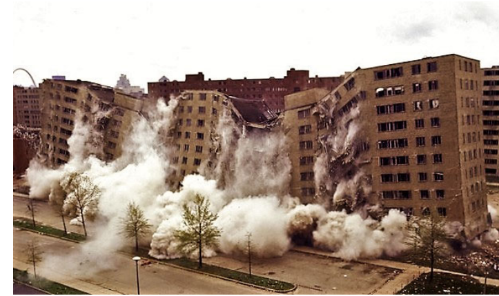
Some structures need to be demolished
